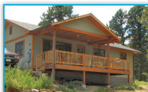
7/3/2007 Completed 10th Home in Estes Park
