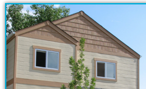
8/30/2009 Completed 42nd home. First Home in Dacono
